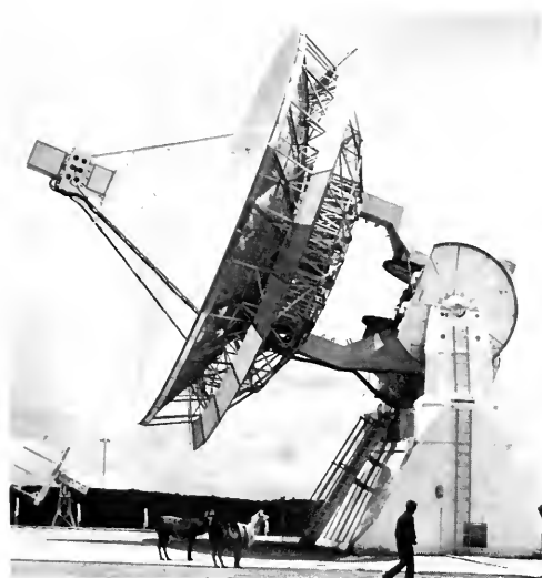
FIGURE 7-23.—The STADAN 12-meter (40-ft) telemetry receiving antenna at Quito, Ecuador.
